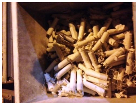
Figure 2: Waste LiFePO 4 batteries in a poor storage arrangement
