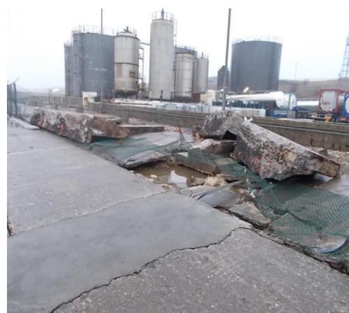
Picture of the damaged wave guard
